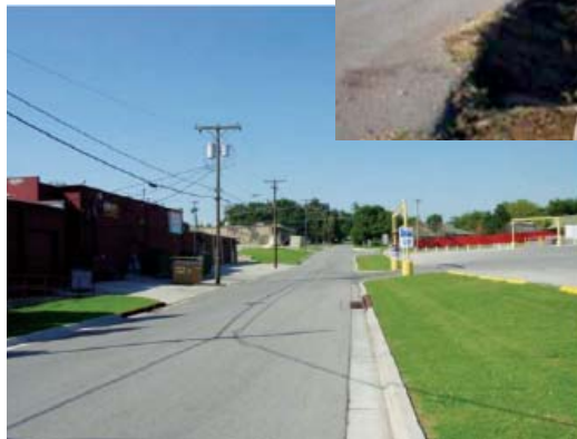
Before and After photos of a recent non-arterial roadway rehabilitation project of S Tacoma Avenue, Tulsa, OK.
