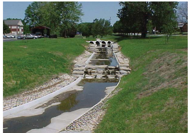
Top: Methodist Manor Detention Facility. Bottom: Methodist Manor Channel Improvements Project.
